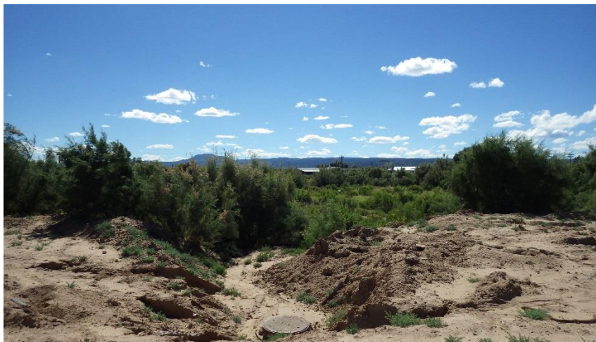
GPP11, salt cedar and erosion along levee road.
