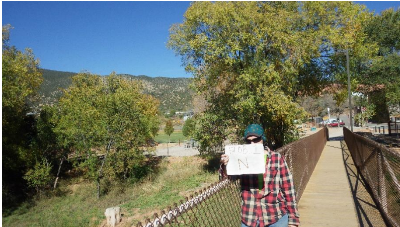
Tijeras Creek 17.08_1_N View facing north inside of polygon 5. Taken from the bridge.
