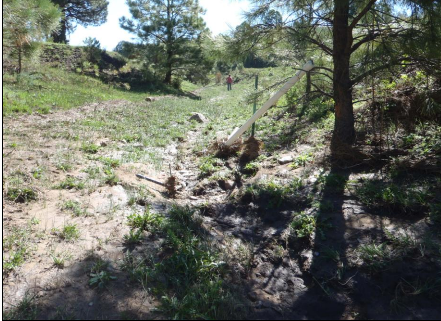
Figure 4.2. The Chilili piezometer in the fall of 2011 after a storm event destroyed the gauge, view facing downstream. The height of the high waterline of this event was determined by the accumulation of debris on the stream banks and within vegetation.
