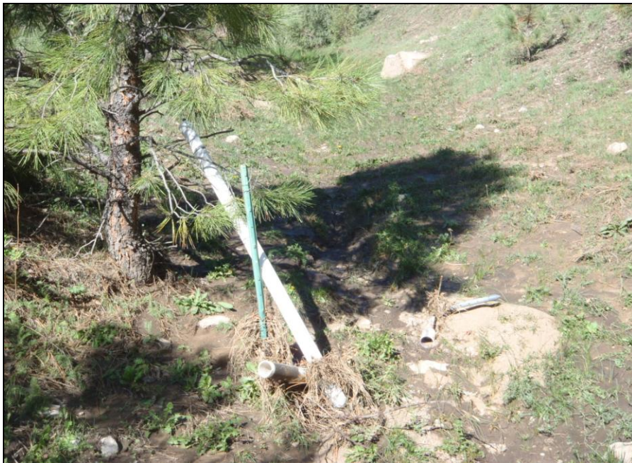
Figure 4.3. The Chilili piezometer in the fall of 2011 after a storm event destroyed the gauge, view facing upstream. The height of the high waterline of this event was determined by the accumulation of debris on the stream banks and within vegetation.
