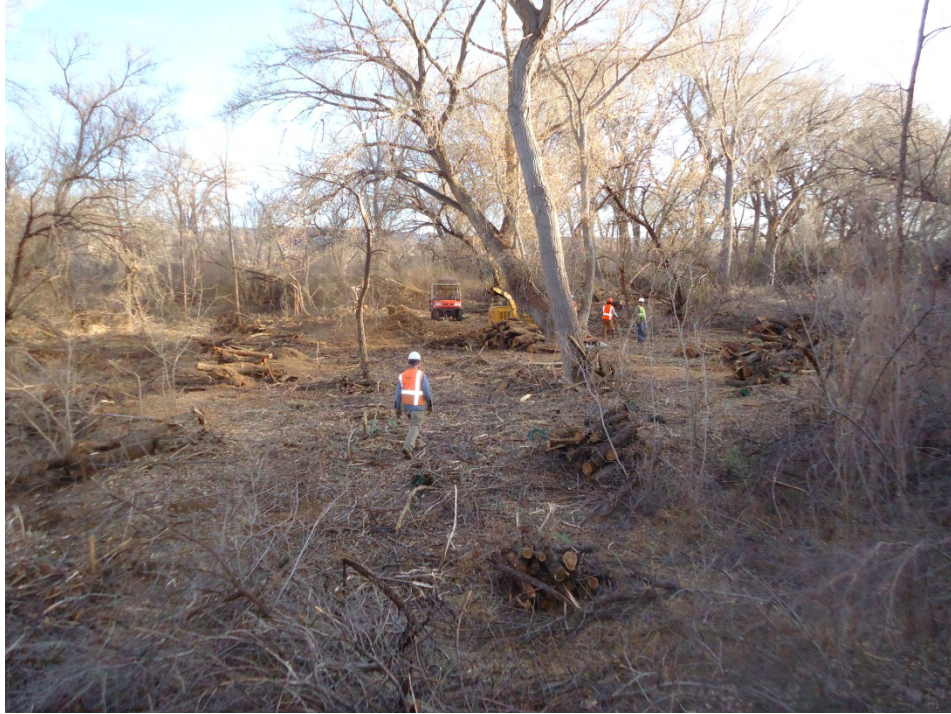
Site during work
