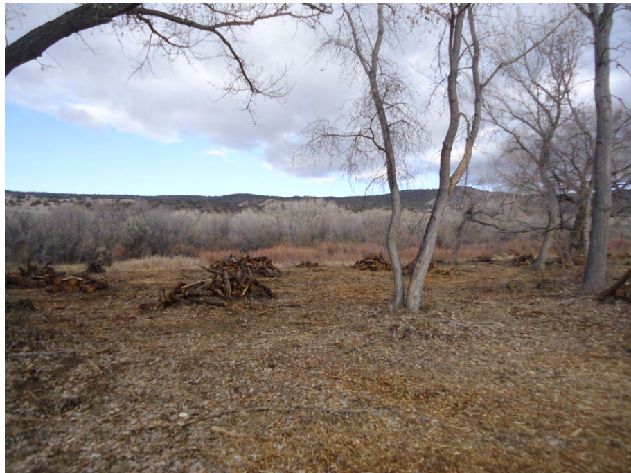
Completed area in southern portion of site
