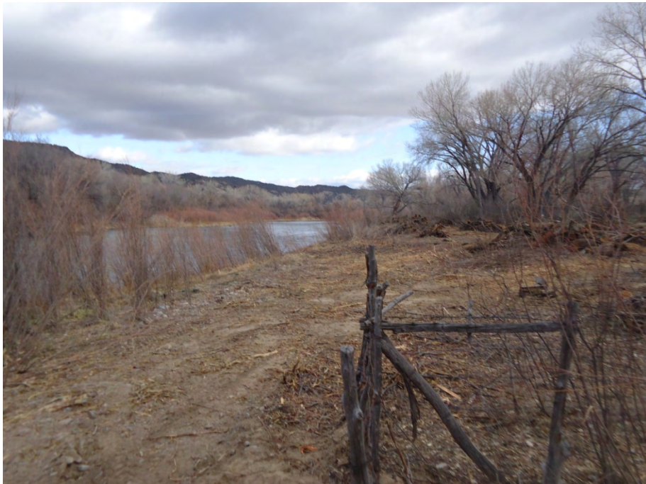
Point 3- After work from gate (looking north)
