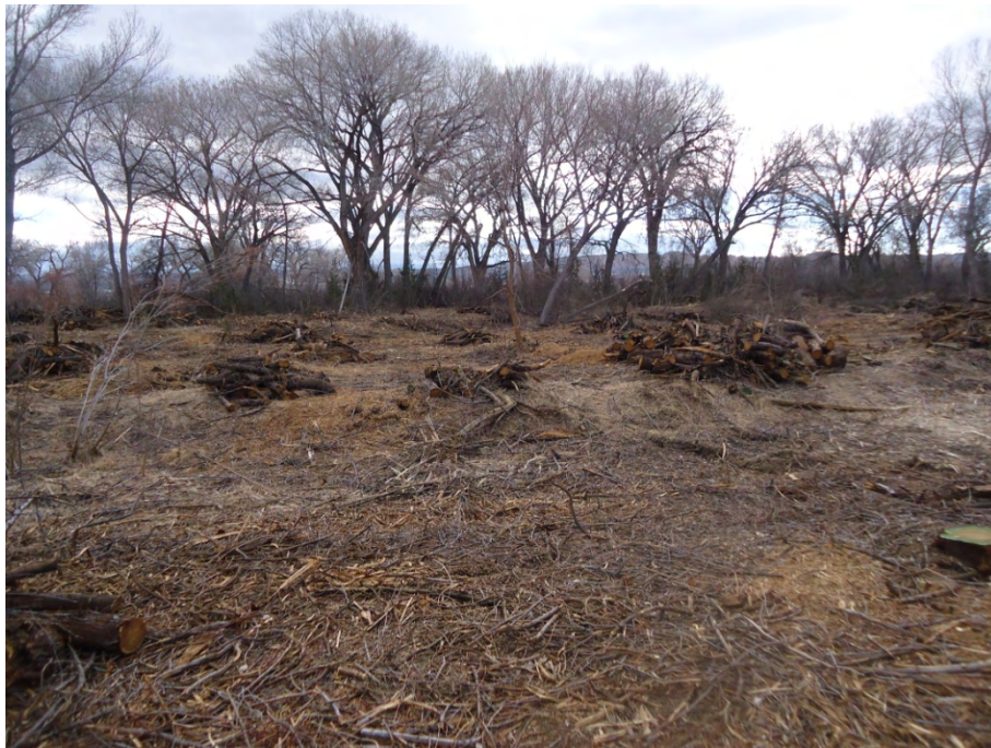
Completed area in southern portion of site
