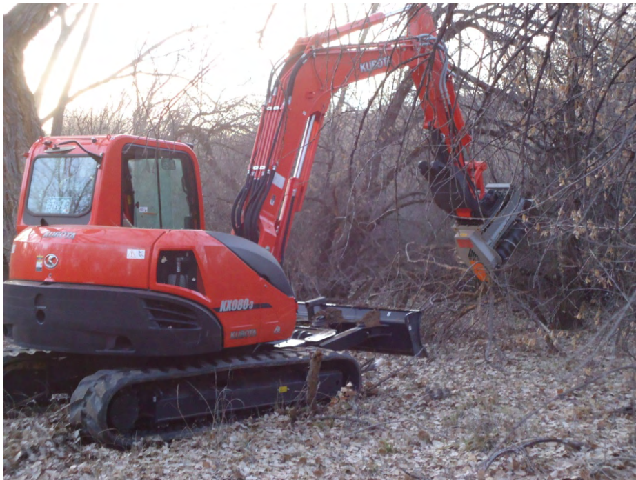
Excavator and FAE mastication head
