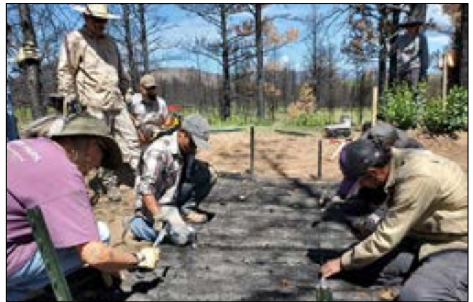
Jeremiah Martin, restoration specialist, teaches workshop attendees how to use burned logs to build an erosion control structure. It was one of 12 free, post-fire workshops hosted by the NMFWR. Photo by Staci Matlock
