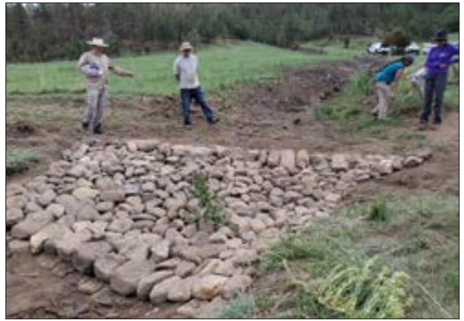
Jeremiah Martin and volunteers discuss a rock structure designed to slow flood waters and reduce erosion. Photo by Kathryn Mahan
