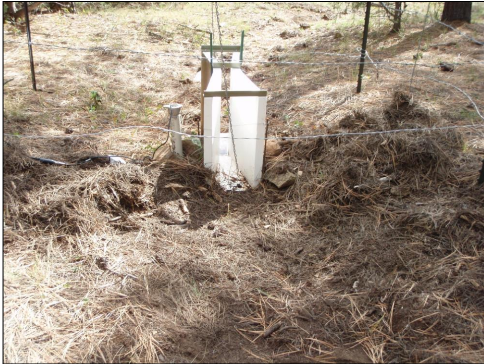
Figure 2.23. Parshall flume located at Chilili site plot 1.
