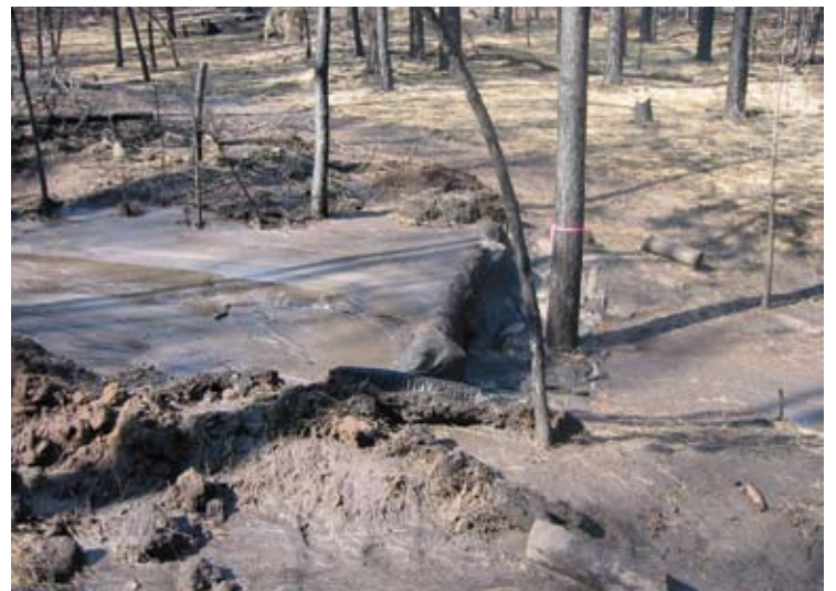
Trash rack and silt dam before (above) and after (right) first thundershower following fire.
