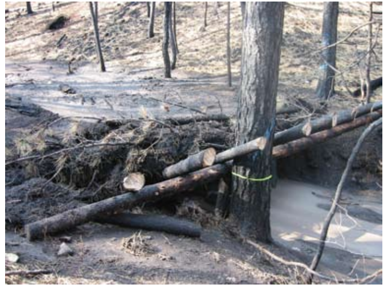
Lower retention dam after first thundershower following fire (no spillway overflow).
