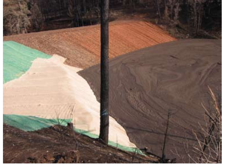
Lower retention dam after first thundershower following fire (no spillway overflow).
