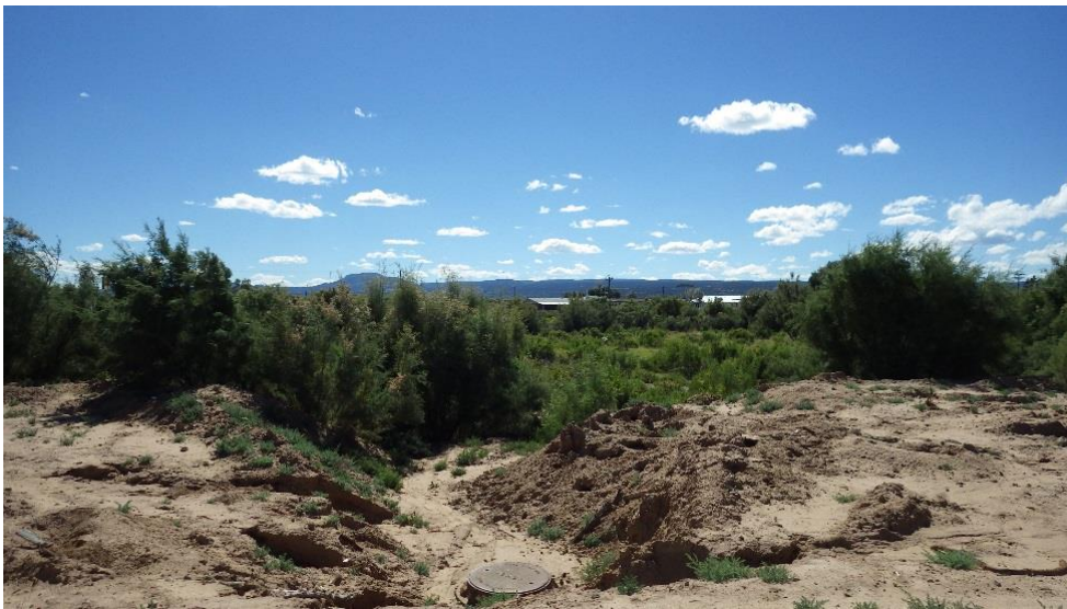
2015: GPP11, salt cedar and erosion along levee road.
