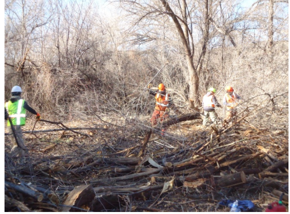
Site During Work
