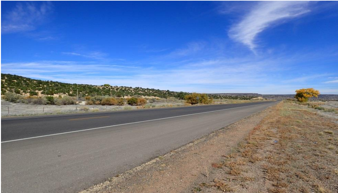
2015: 16.13_2_N W. View facing north- west.
