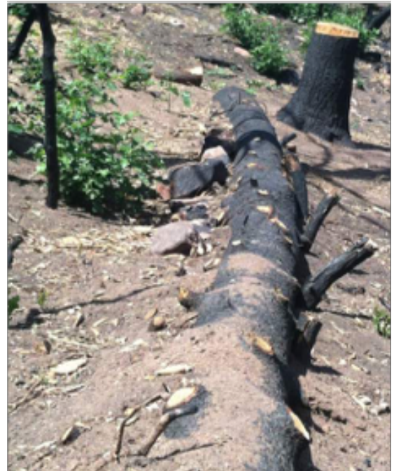
Figure 4. Example of stakes, stump, and backfilling for contour log felling (Coalition for Upper South Platte, 2015).
